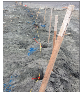
6. Tie off knot (we recommend a double wrap clove hitch)
