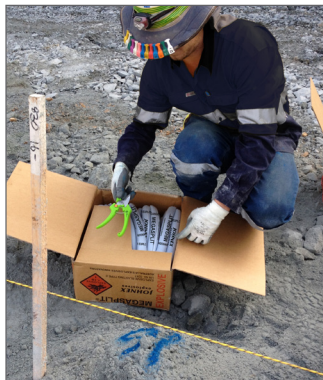
1. Lay out explosives along line of drilled pre-split holes. Boxes should be laid out upside down.
