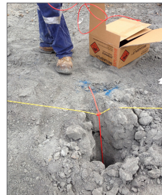
7. Cut off excess detonating cord.
