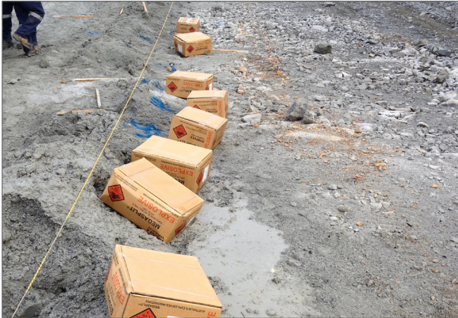
1. Lay out explosives along line of drilled pre-split holes. Boxes should be laid out upside down.
