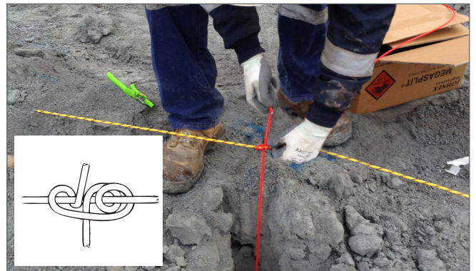
6. Tie off knot (we recommend a double wrap clove hitch)
