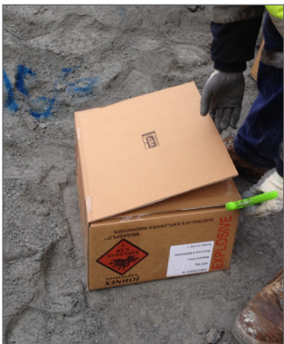
2. Open box to expose base charge.
