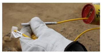
2. Feed the detonator fully through the cord tunnel.
